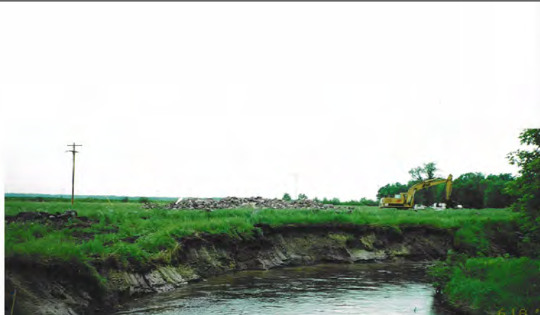
Site A Before Construction, Bank Slumping
