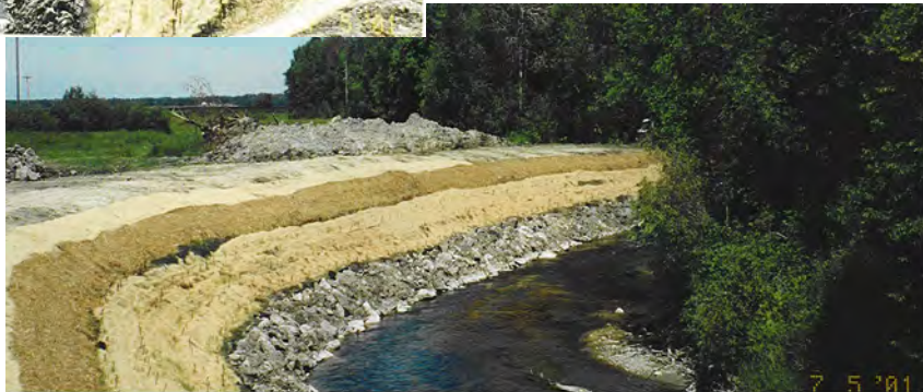
Bank Stabilization Site B Willows Shortly After Construction
