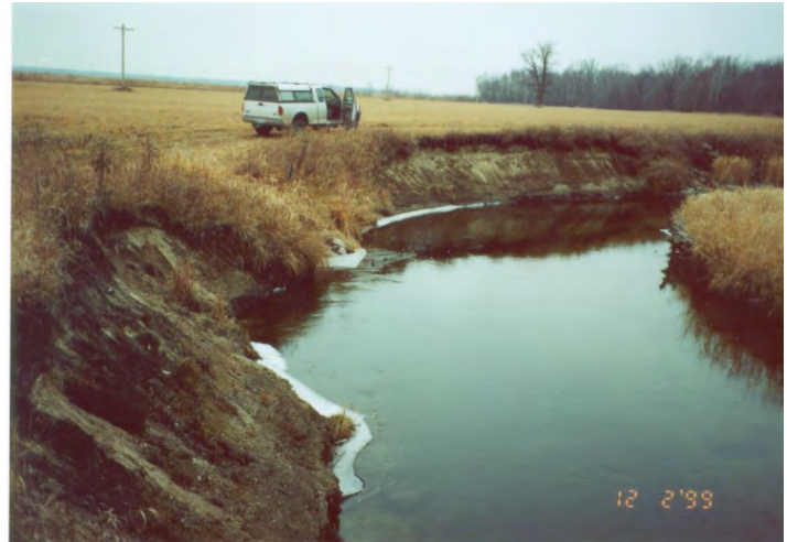
Site A Before Construction, Bank Slumping
