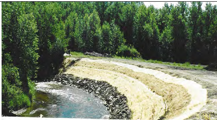
Bank Stabilization Site B Willows, Fiber Blanket, and Riprap Around Bend
