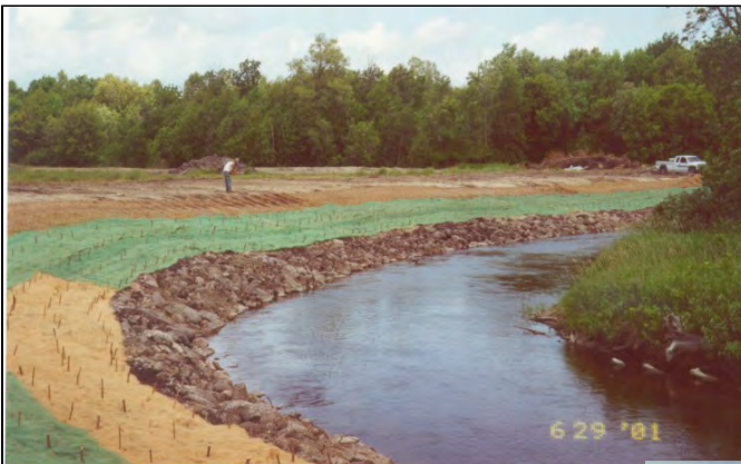
Bank Stabilization Site A Willows and Riprap Along Bend
